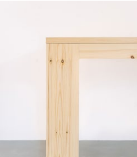
Front view of the leg-top joint,
